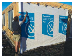
Fix Watergate Plus securely to the frame.
